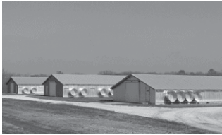
APPLIED BROILER RESEARCH UNIT (SAVOY) - These four full-sized broiler houses are equipped with computerized environmental control and data collections systems capable of commercial-type production research.
